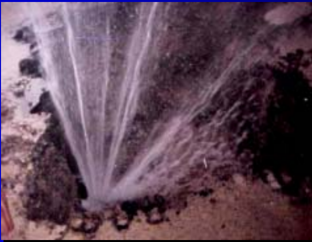
Water leakage at a domestic intake
